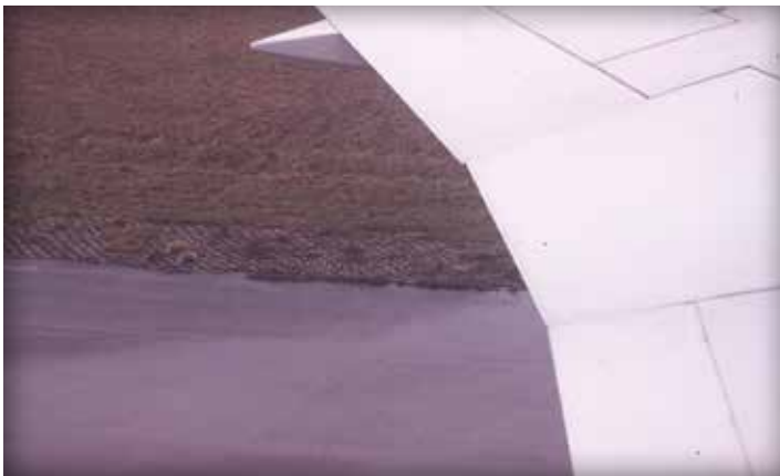
Figure 11. Airfield taxiway shoulder
