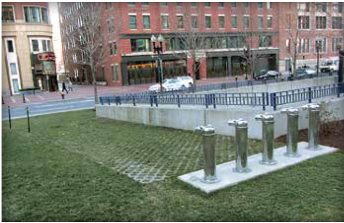
Figure 7. Emergency access lane for fire trucks
