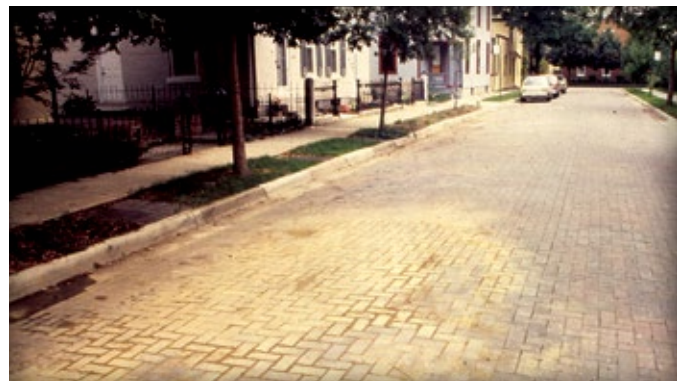
Figure 5. The final paver surface is continuous. There are no cuts or damage to the pavement.
