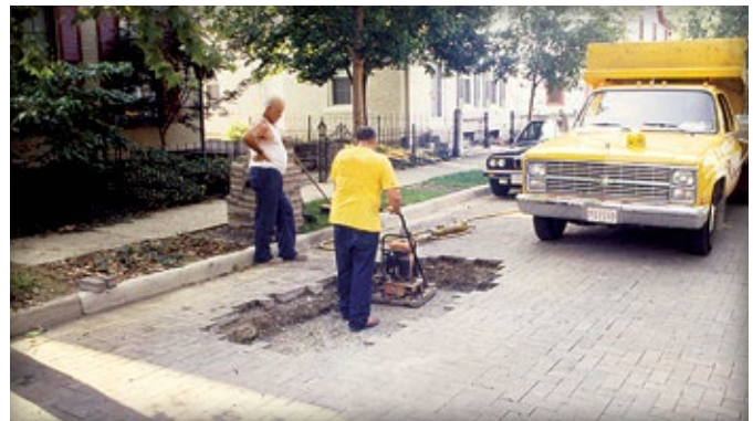
Figure 3. Compaction of the base
