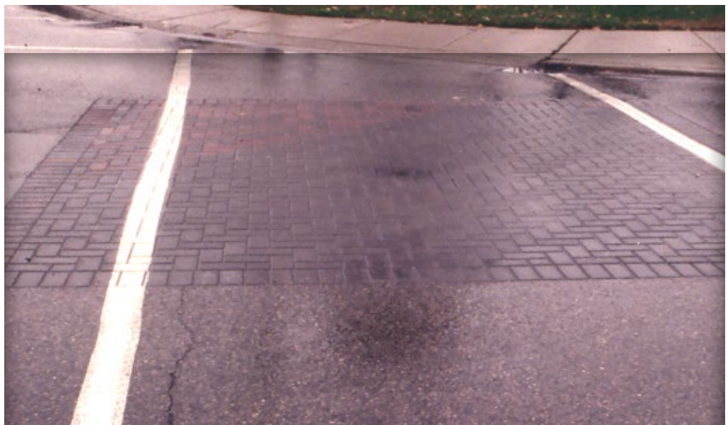
Figure 13. Concrete pavers in utility cuts can be painted as any other pavement.
