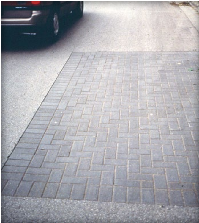
Figure 8. Utility cut repair in a residential area in London, Ontario.
