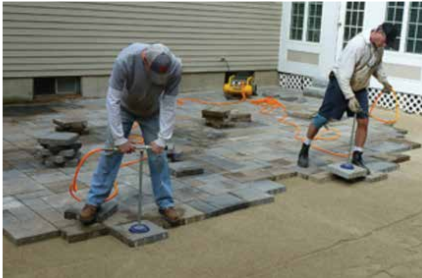
Figure 15. Using vacuum equipment to install paving slabs in a residential application
