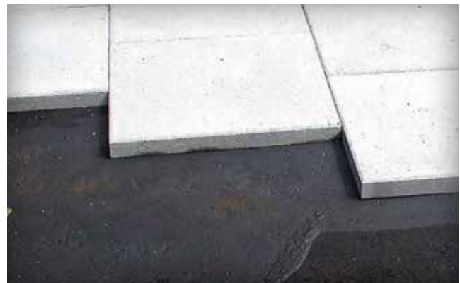
Figure 7. Sidewalk application illustrating the neoprene adhesive on an asphalt bedding layer under paving slabs
