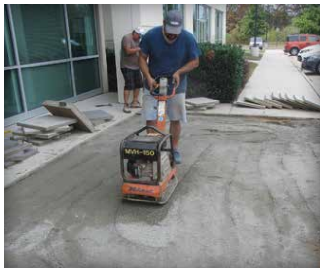
Figure 5. Precompacting the bedding sand
