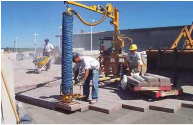
Figure 11. Self-contained vacuum lifter with boom
