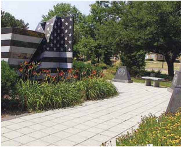
Figure 14. High SR paving slabs
