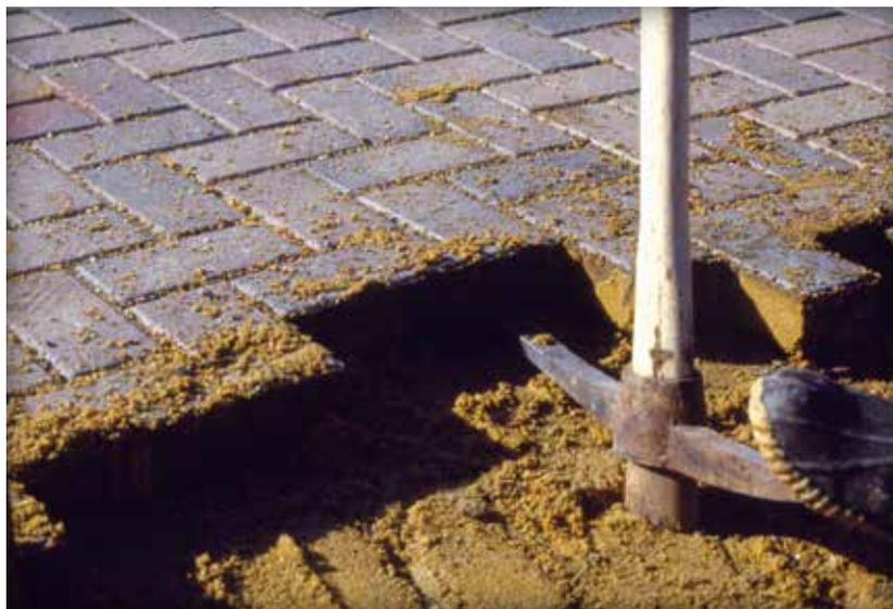
Figure 6. Prying out the remaining pavers
