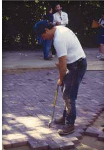
Figure 13. Adjusting joint spacing and alignment.
