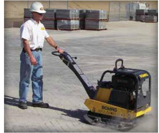
Figure 14. Second and final compaction of the pavers. The first compaction occurs after the pavers are placed (no sand in the joints). The second compaction works the sand on pavers into the joints. This process causes the pavers to interlock.
