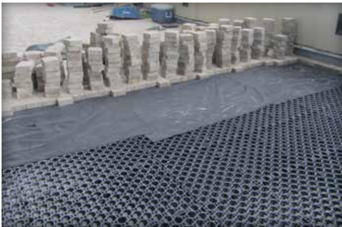
Figure 7. Concrete pavers on geotextile over plastic grids
