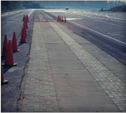
Figure 5. The test track section and concrete paver surface at The Pennsylvania Transportation Institute test facility.
